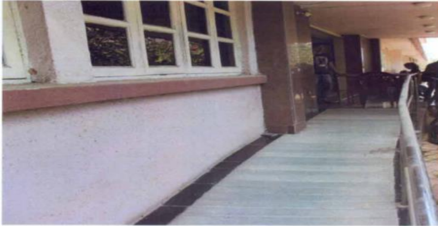
Fig.3 Ramp to enter the Institute building
